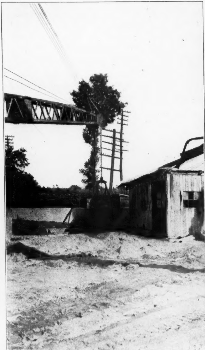
Derrick Removing Mud from Settling Pond
